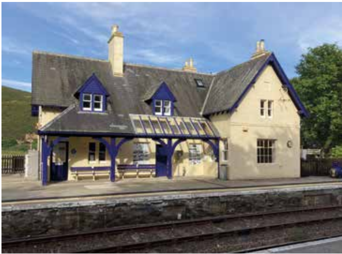
Fig.4: Helmsdale Station. Author's photograph.
